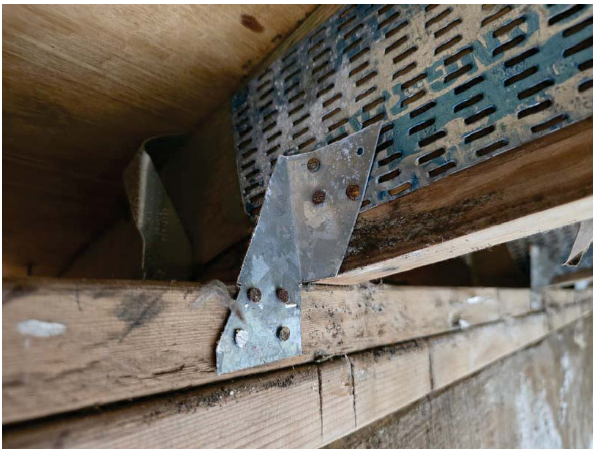
ROOF TO WALL - HURRICANE CLIPS - OK
