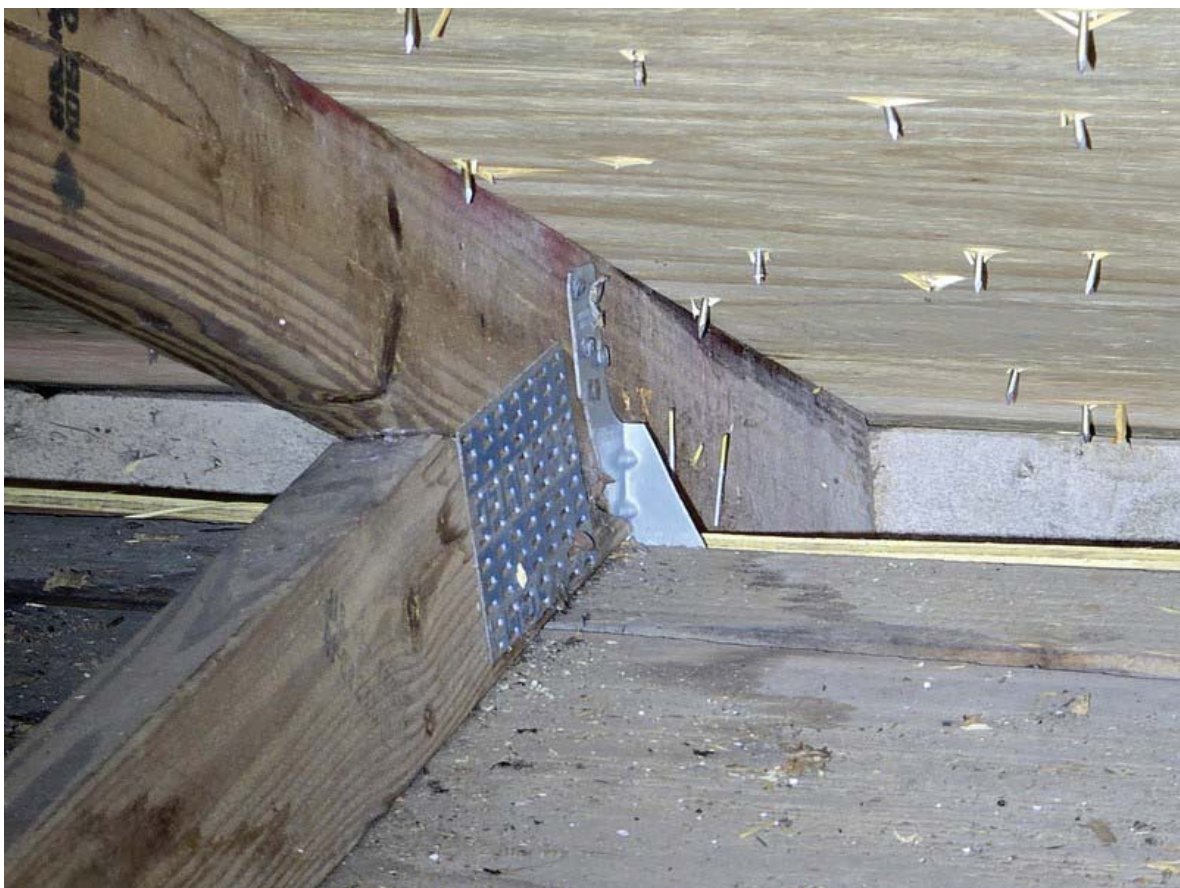
ROOF TO WALL - HURRICANE CLIPS - OK
