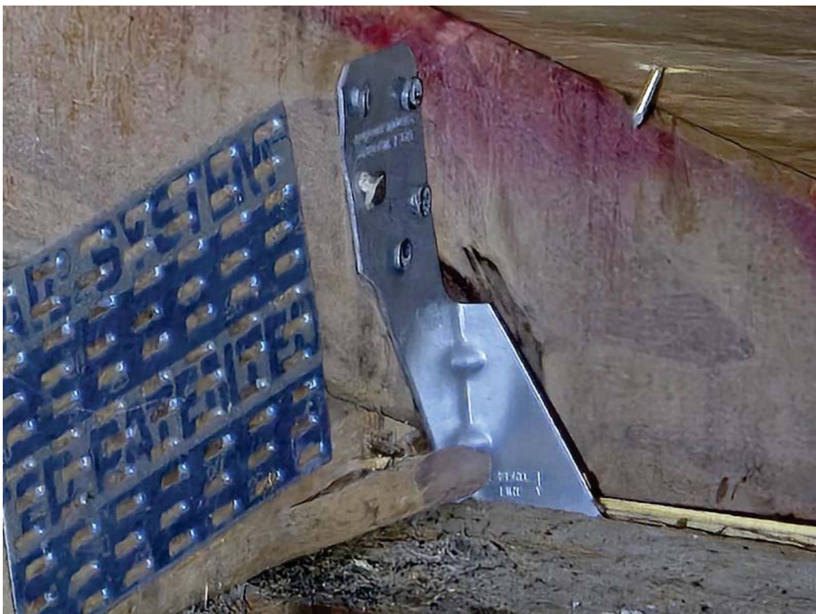
ROOF TO WALL - HURRICANE CLIPS - OK
