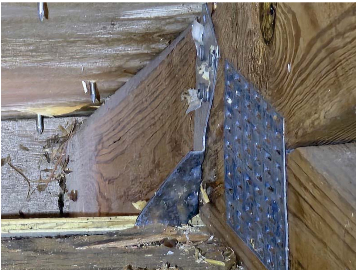
ROOF TO WALL - HURRICANE CLIPS - OK
