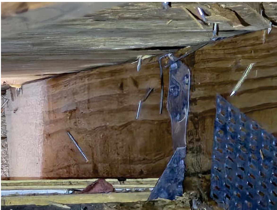
ROOF TO WALL - HURRICANE CLIPS - OK
