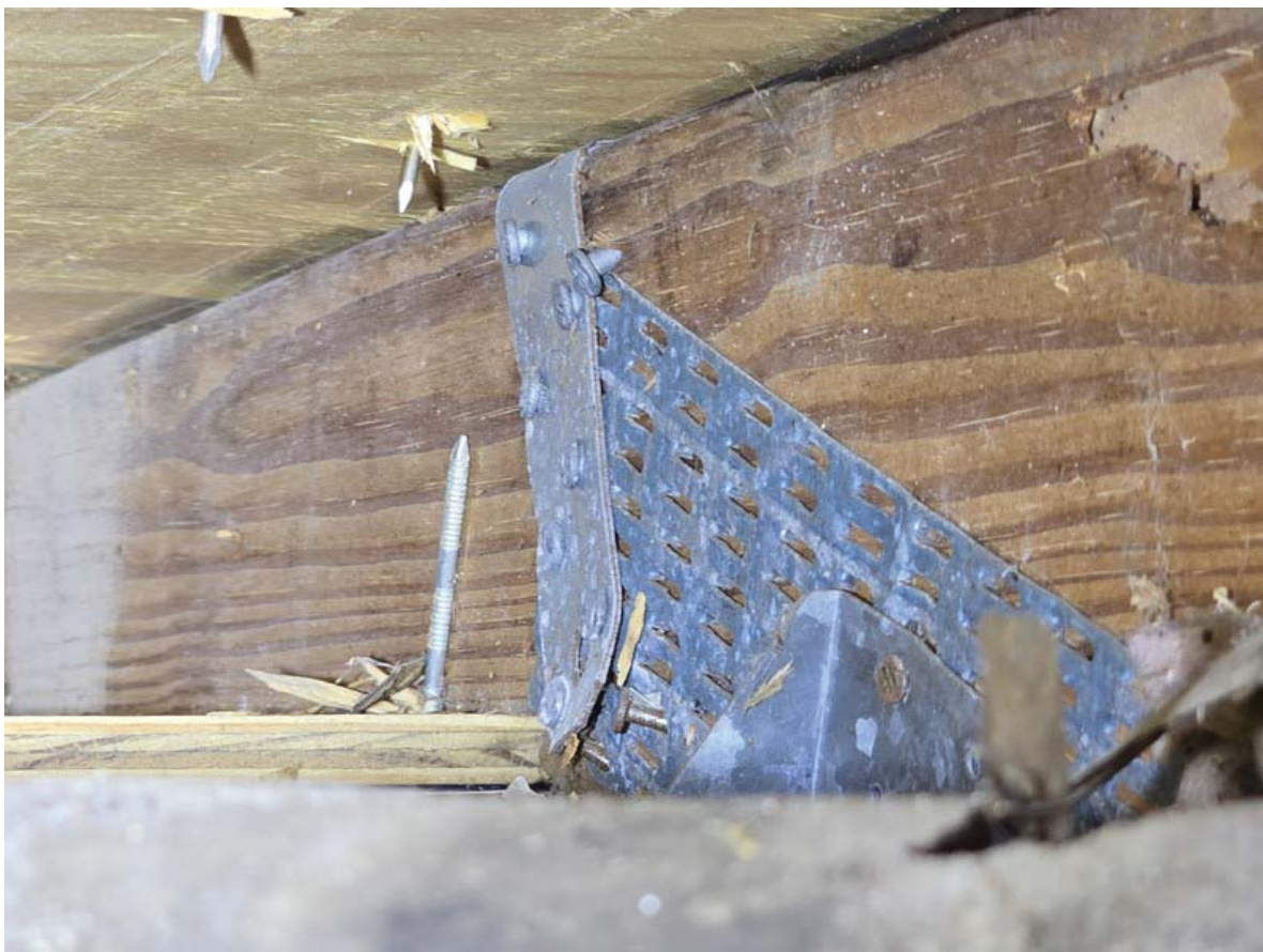
ROOF TO WALL - STRAPS BACK SIDE - OK
