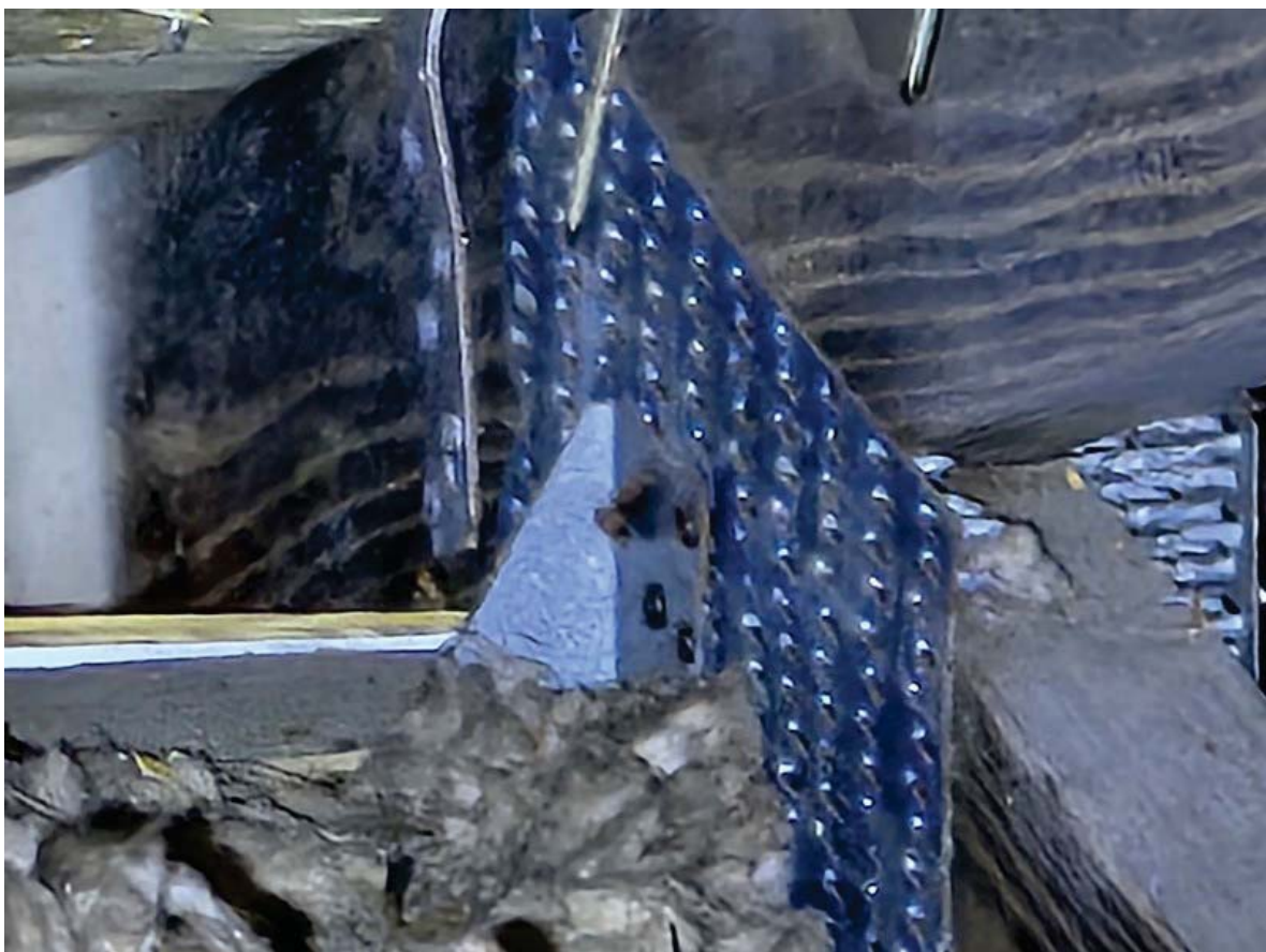
ROOF TO WALL - HURRICANE CLIPS - OK
