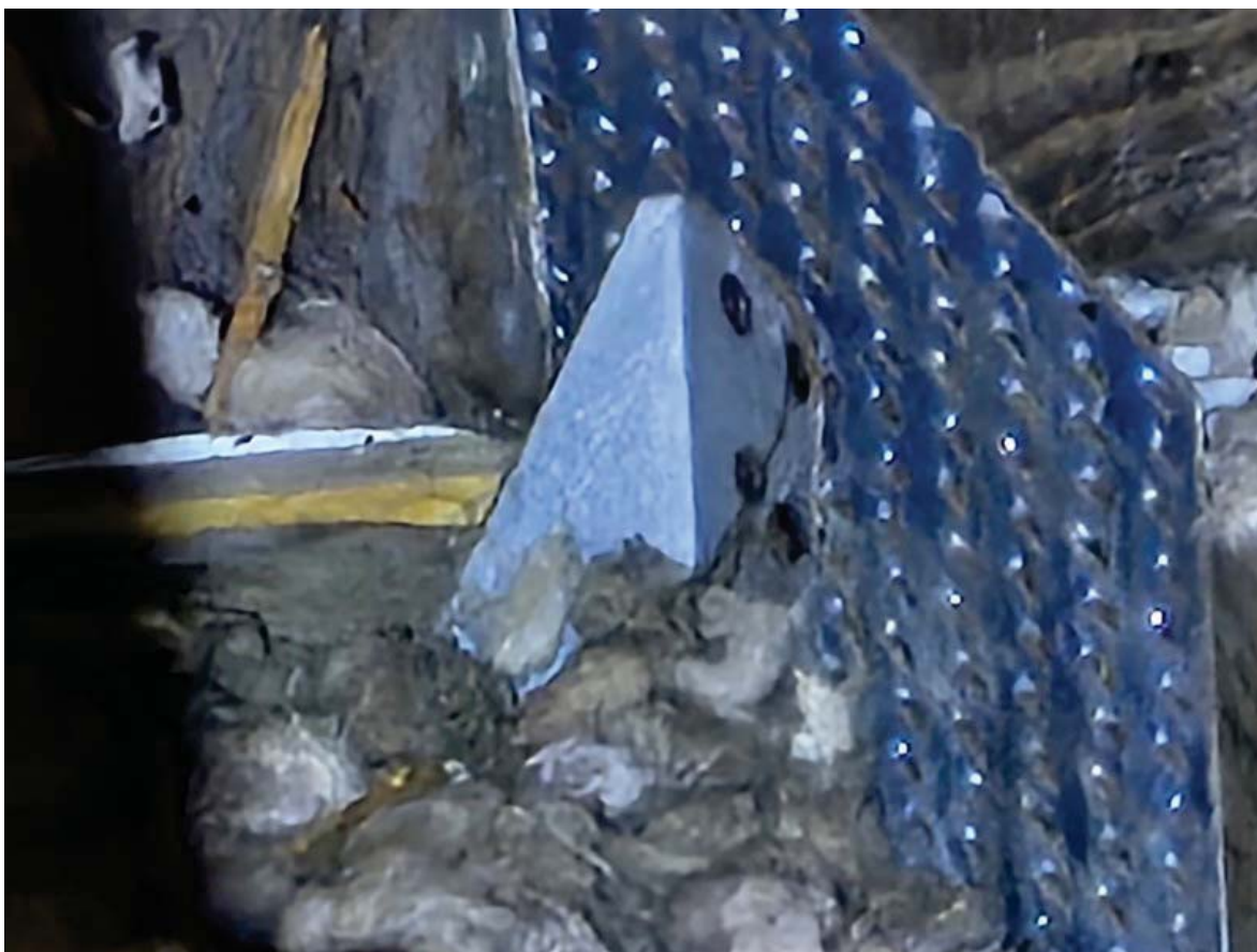
ROOF TO WALL - HURRICANE CLIPS - OK
