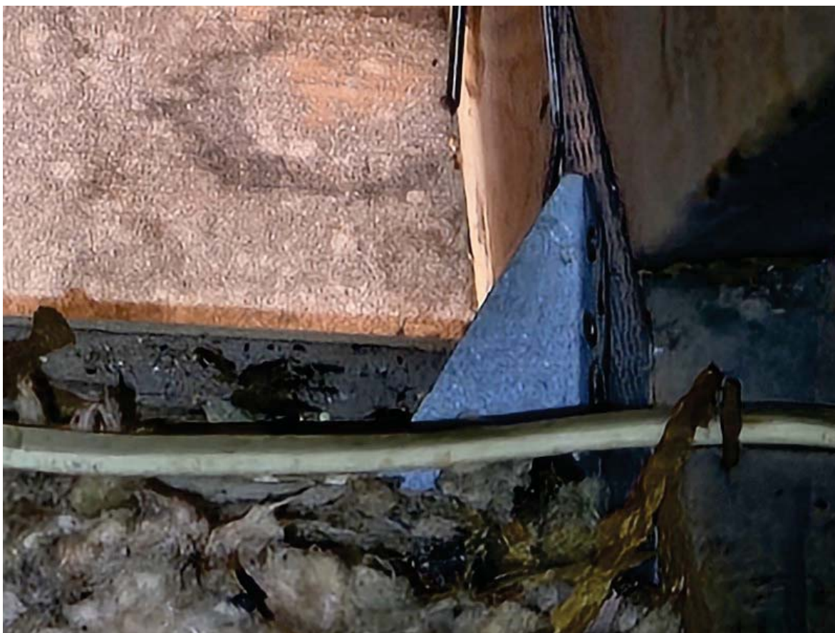
ROOF TO WALL - HURRICANE CLIPS - OK
