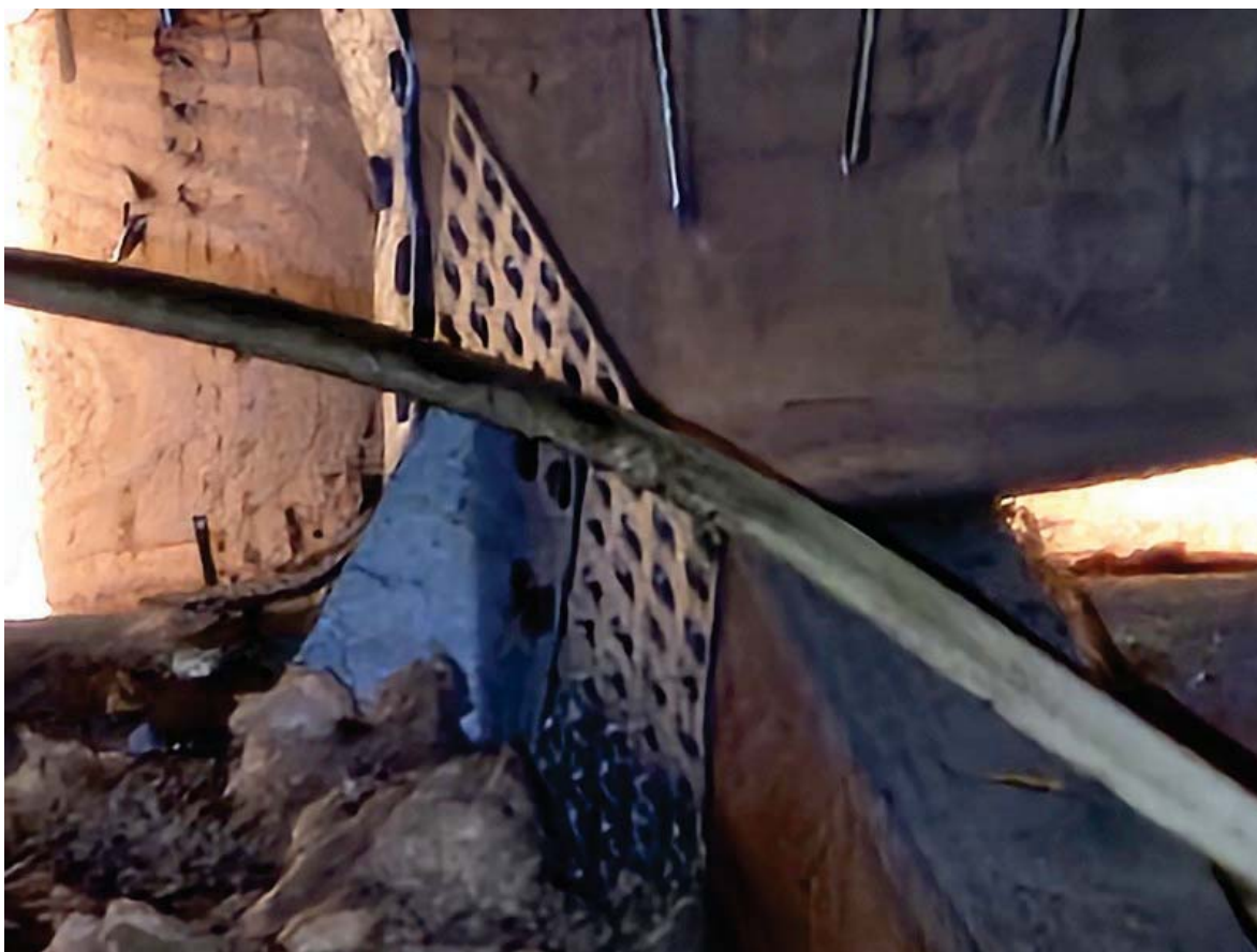
ROOF TO WALL - HURRICANE CLIPS - OK
