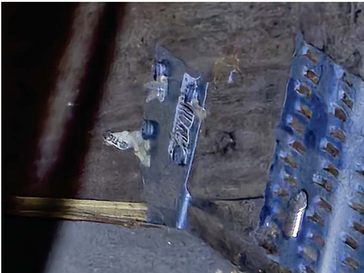
ROOF TO WALL - HURRICANE CLIPS - OK
