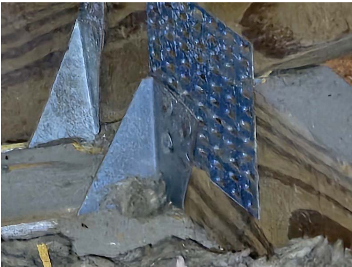
ROOF TO WALL - HURRICANE CLIPS - OK
