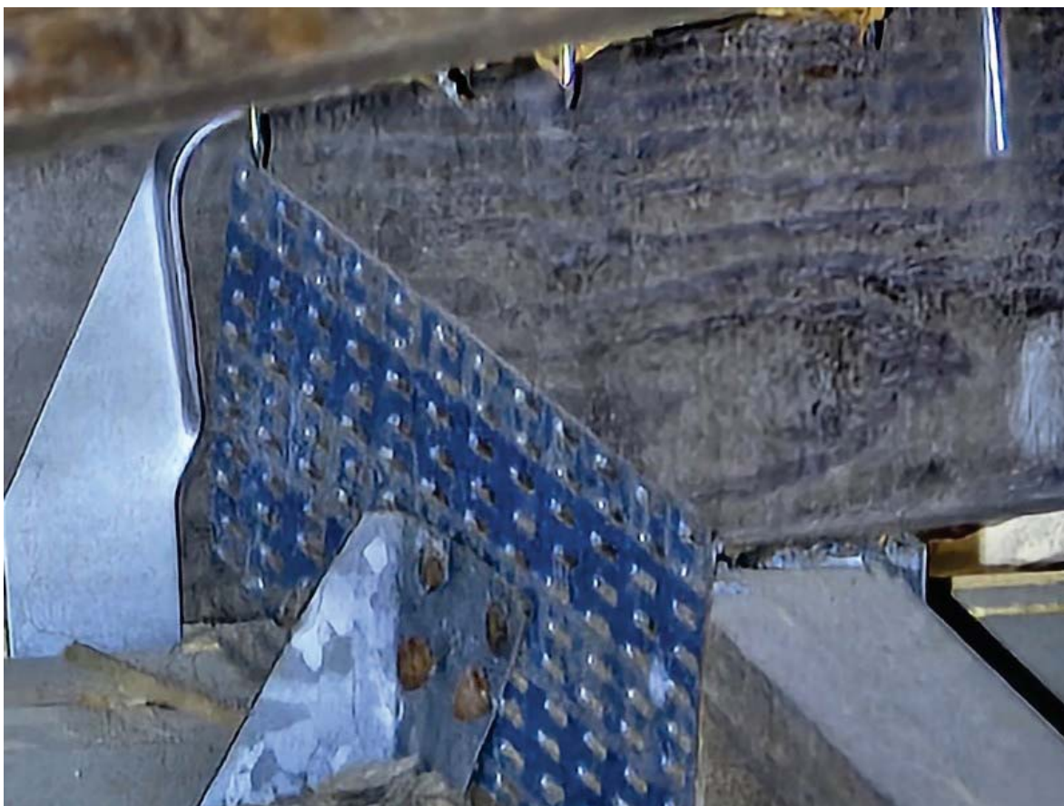
ROOF TO WALL - HURRICANE CLIPS - OK
