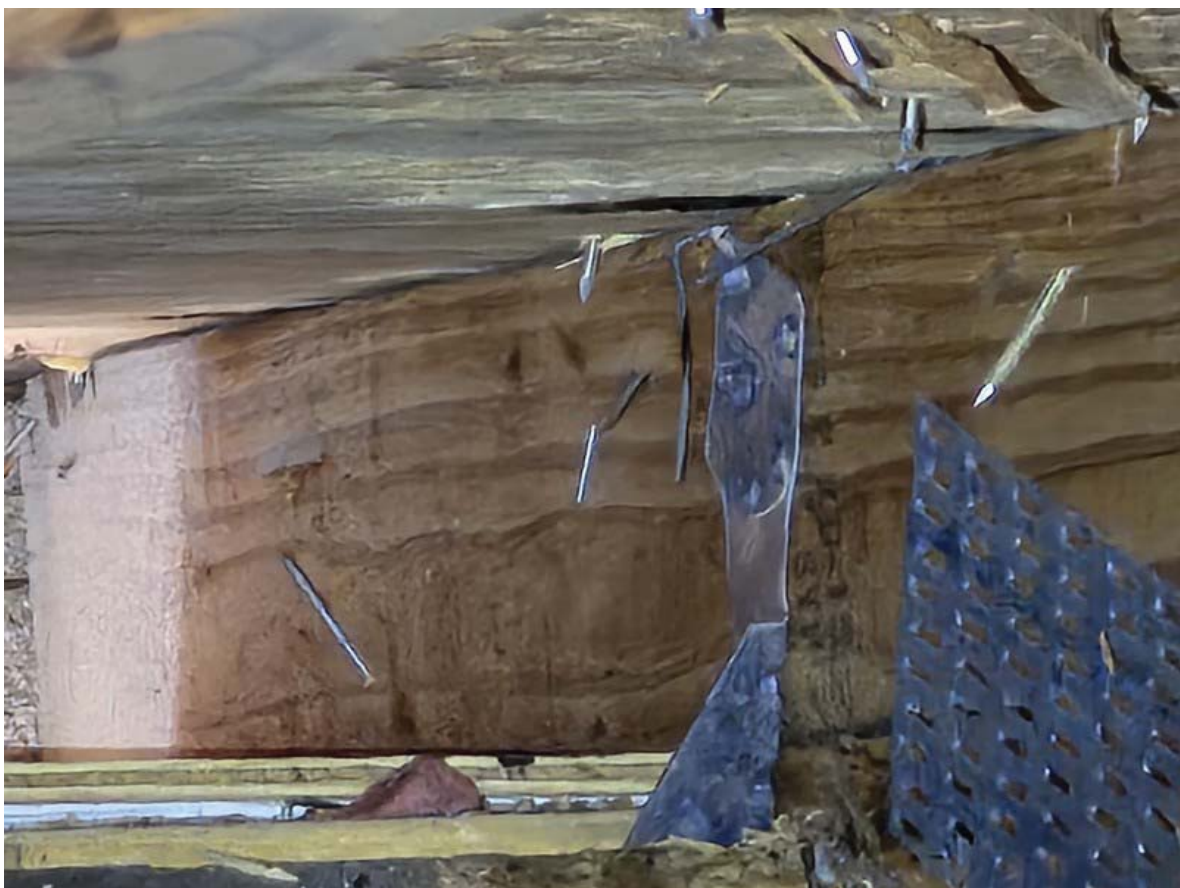
ROOF TO WALL - HURRICANE CLIPS - OK
