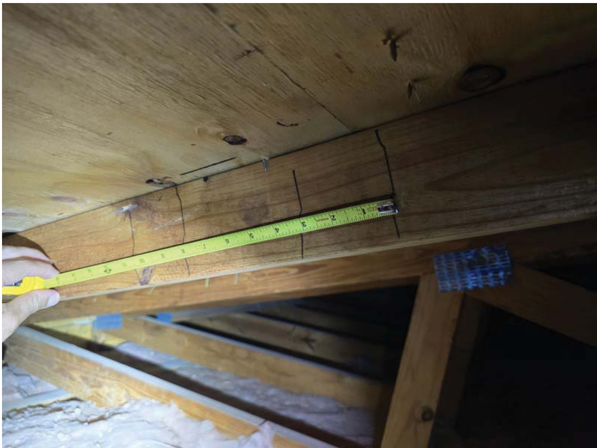
ROOF DECK NAILED EVERY 6" IN FIELD OR BETTER OK
