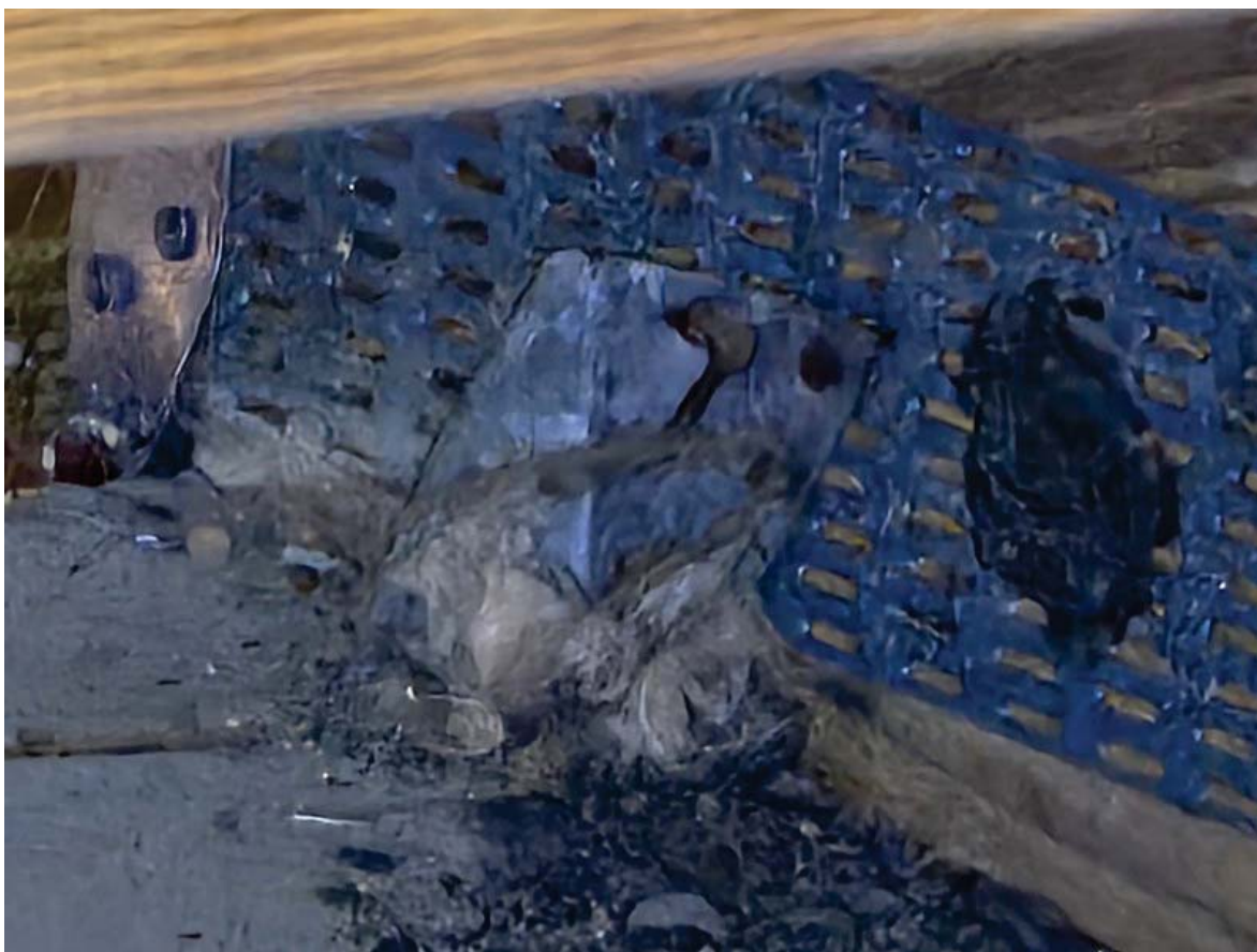
ROOF TO WALL - HURRICANE CLIPS - OK
