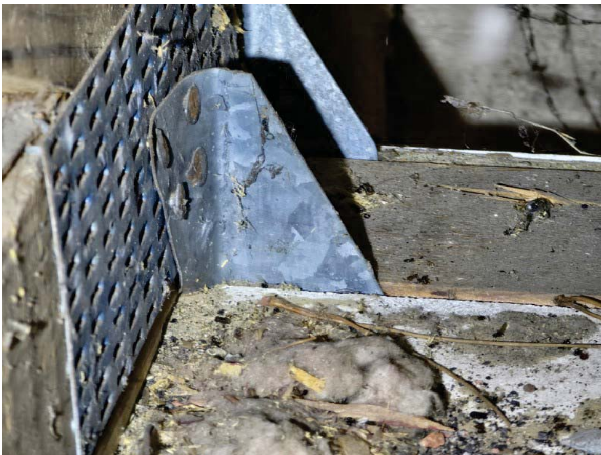
ROOF TO WALL - HURRICANE CLIPS - OK
