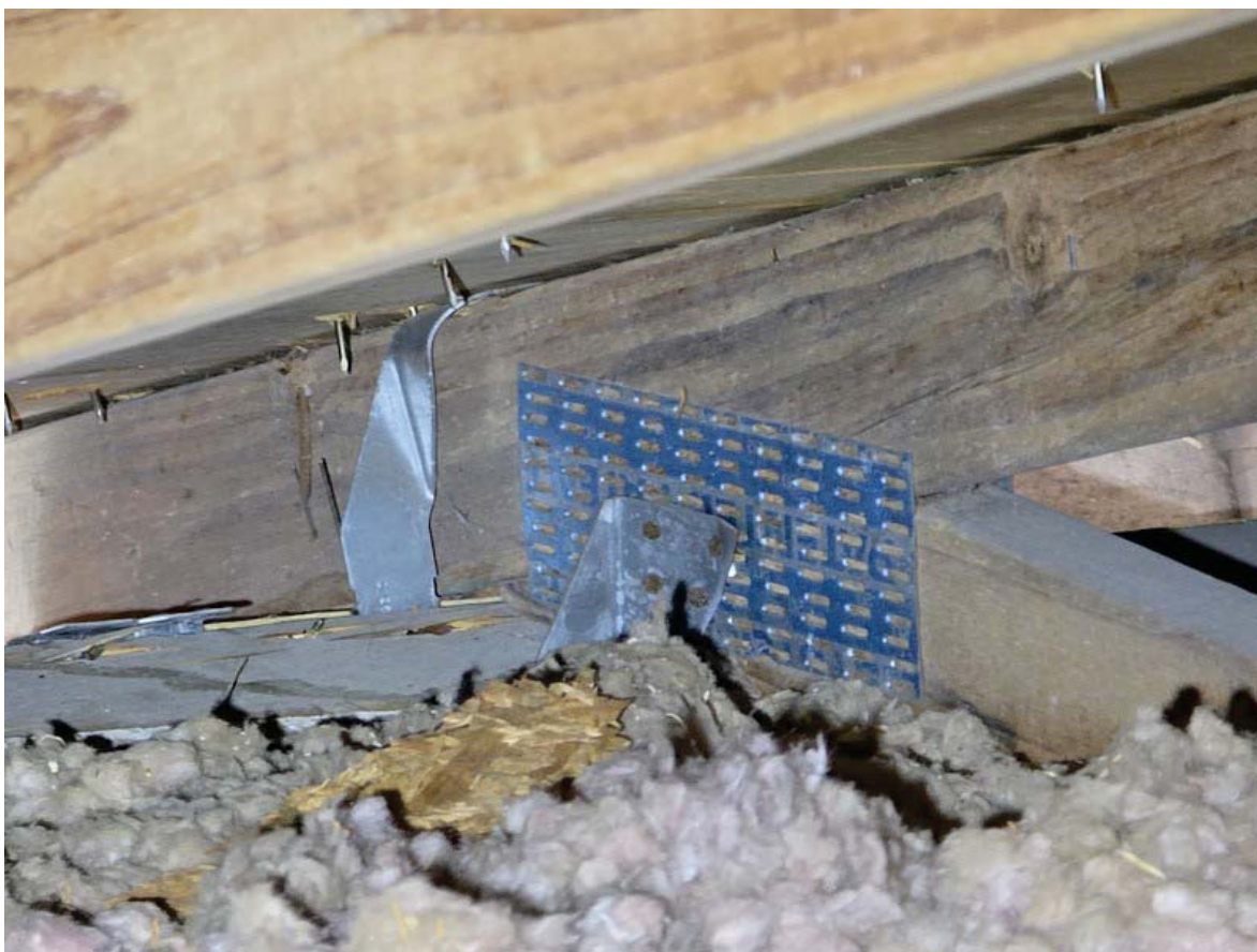
ROOF TO WALL - HURRICANE CLIPS - OK
