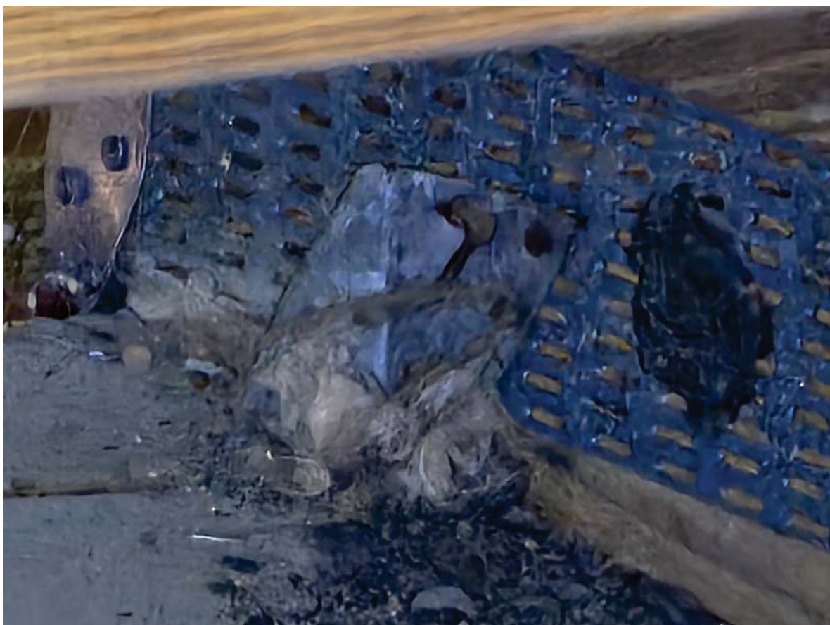
ROOF TO WALL - HURRICANE CLIPS - OK
