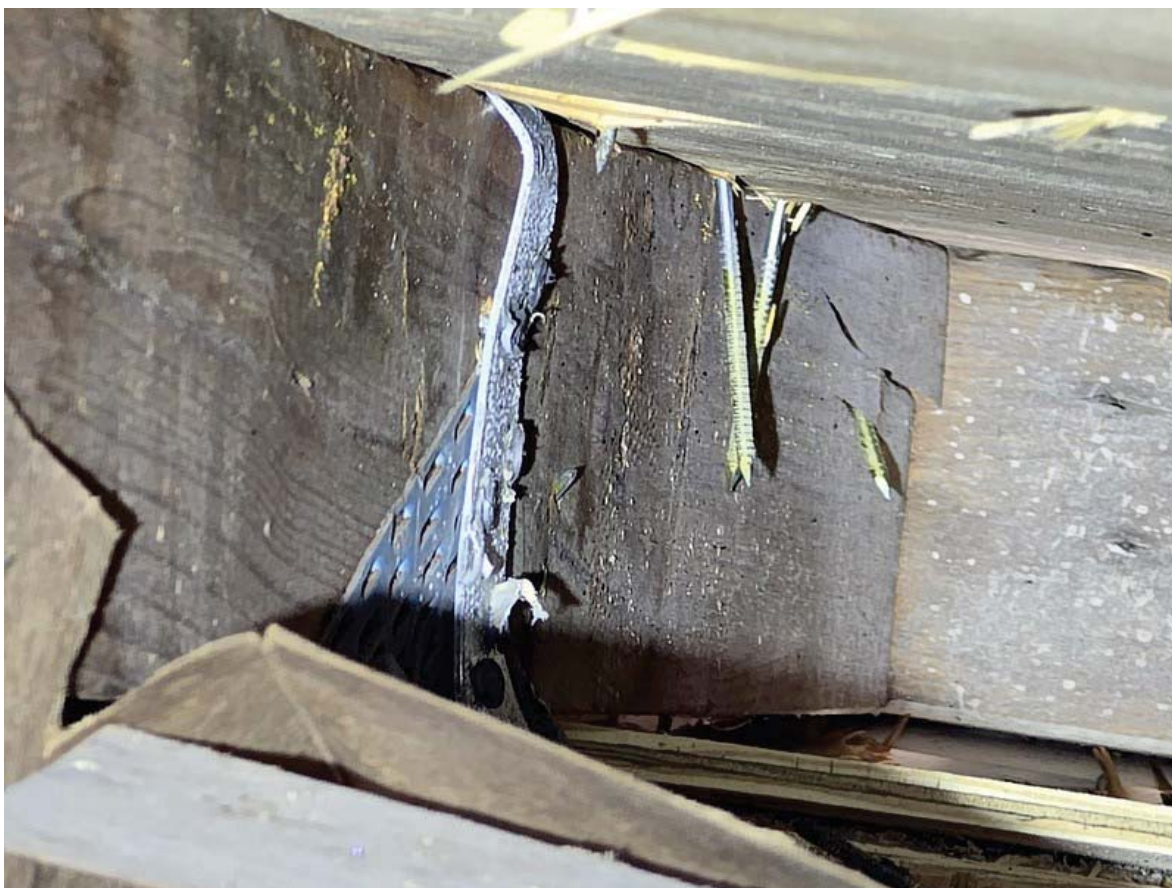
ROOF TO WALL - HURRICANE CLIPS - OK
