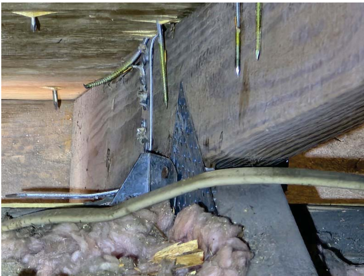
ROOF TO WALL - HURRICANE CLIPS - OK
