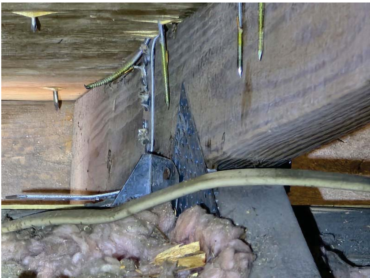
ROOF TO WALL - HURRICANE CLIPS - OK
