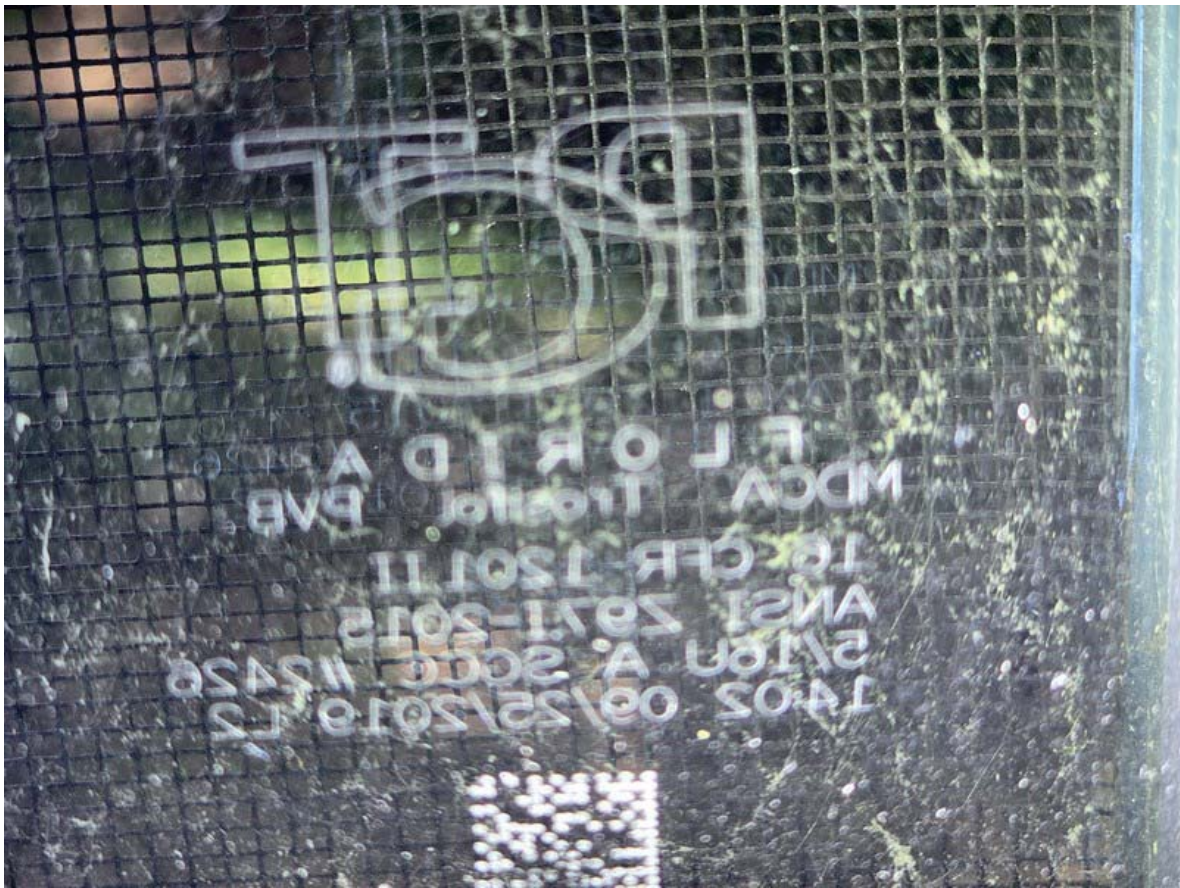
ALL WINDOWS WERE MCDA IMPACT RATED LAMINATED SAFETY GLASS
