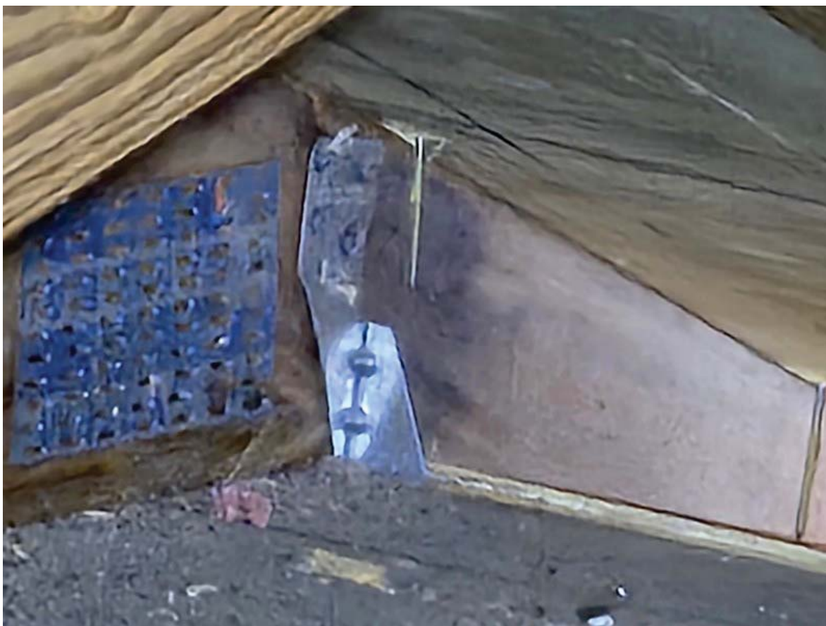
ROOF TO WALL - HURRICANE CLIPS - OK
